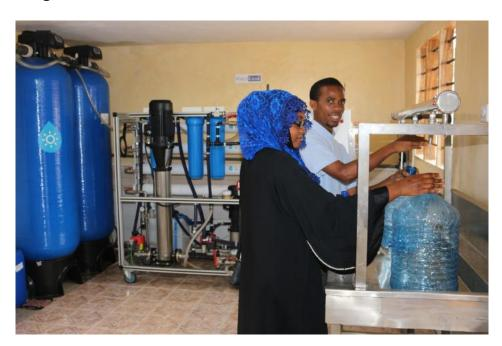
Solar-powered reverse osmosis membrane elements from LANXESS' Lewabrane brand are used in the village Burani; Kenya, to turn raw water with a high salt content of 4,800 ppm into potable water.
